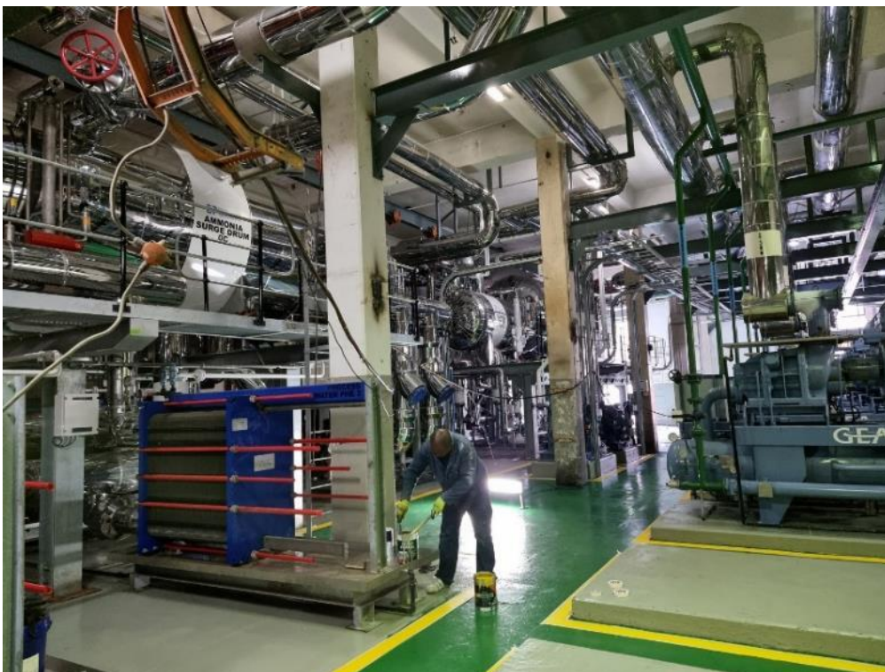
Image 4: CaaS ammonia refrigeration system at a dairy processing plant of Clover, South Africa
