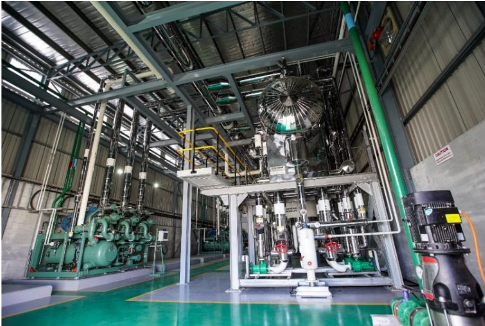
Image 3: CaaS ammonia refrigeration system at a poultry producing plant of Sovereign Foods, South Africa
